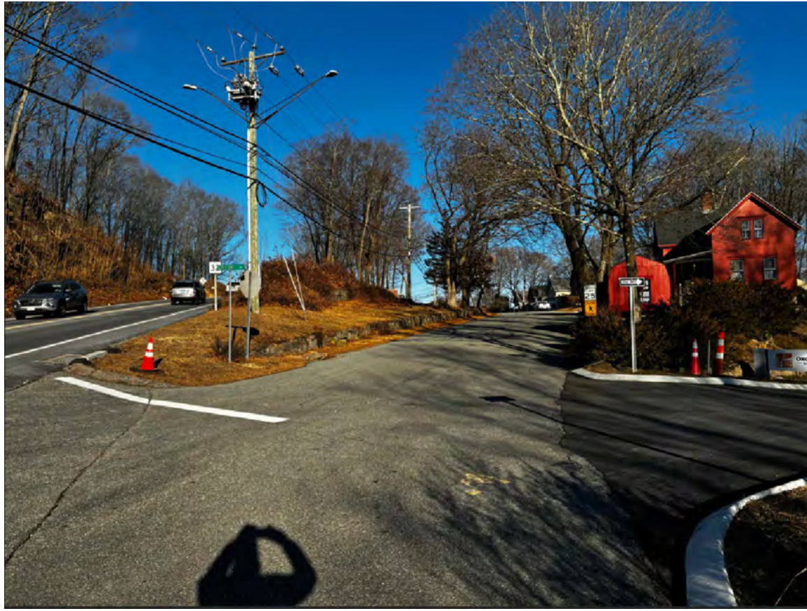
17. View of Crescent Street from RT 32 at Oxoboxo Loft entry. Trail can readily serve this 72 unit affordable housing development.
