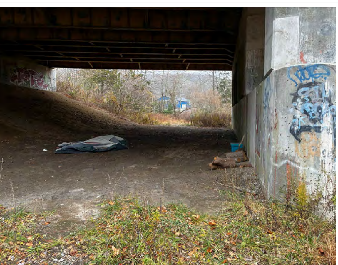
7. View under the I-395 bridge. Space is ample for the path's passage.
