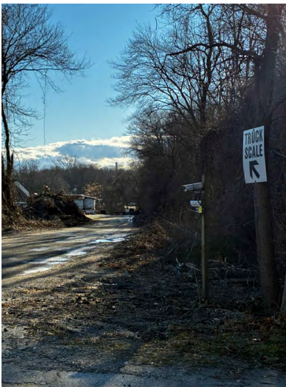
4. View of rail bed looking east; used by local scrap yard. path and uses will require separation; owner engaged in conversation
