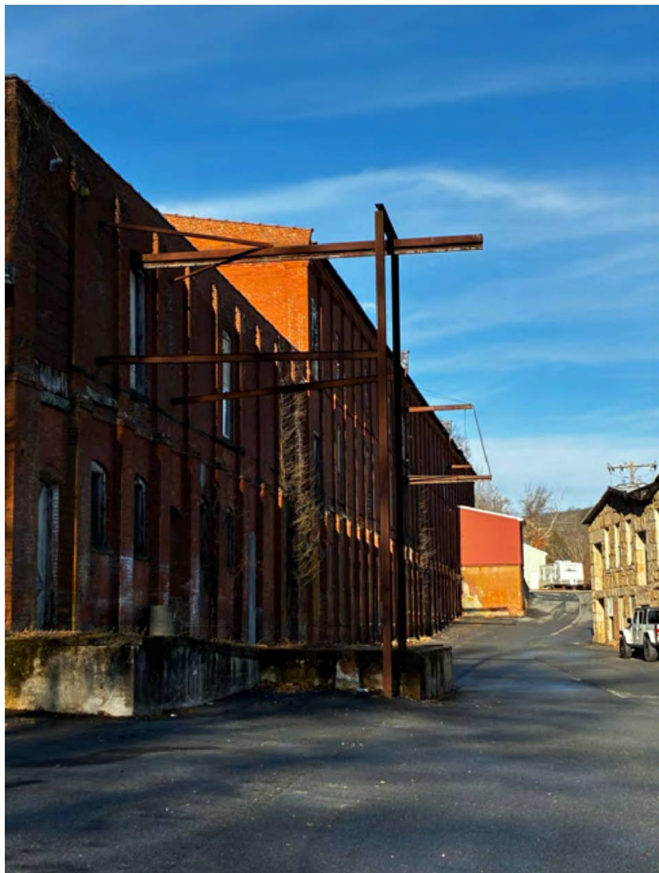
2a. Town owned property subject of 52 residential units. Property will convey trail after redevelopment.
