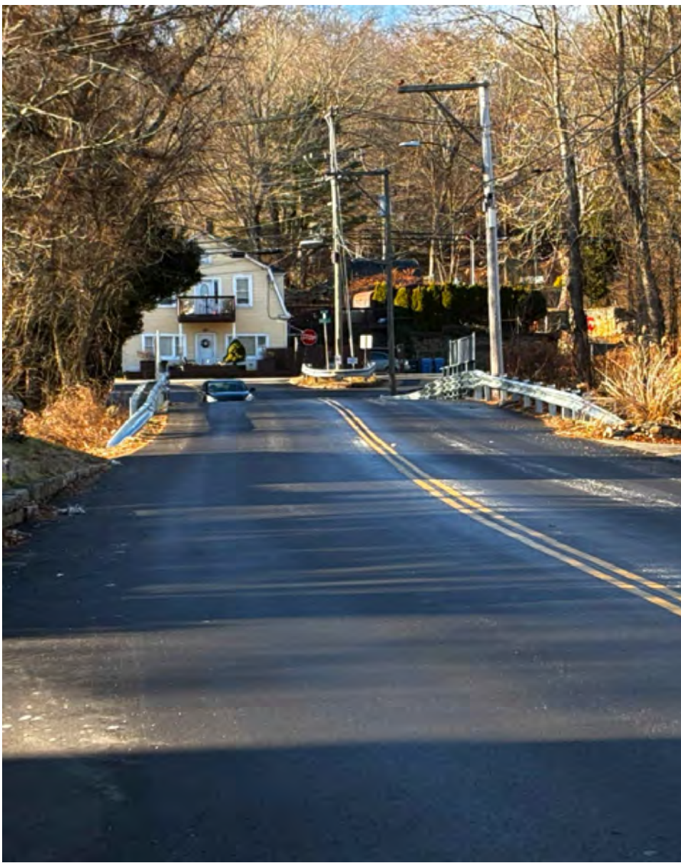
1a. Palmettown: Bridge St looking south, bridge over former rail.
